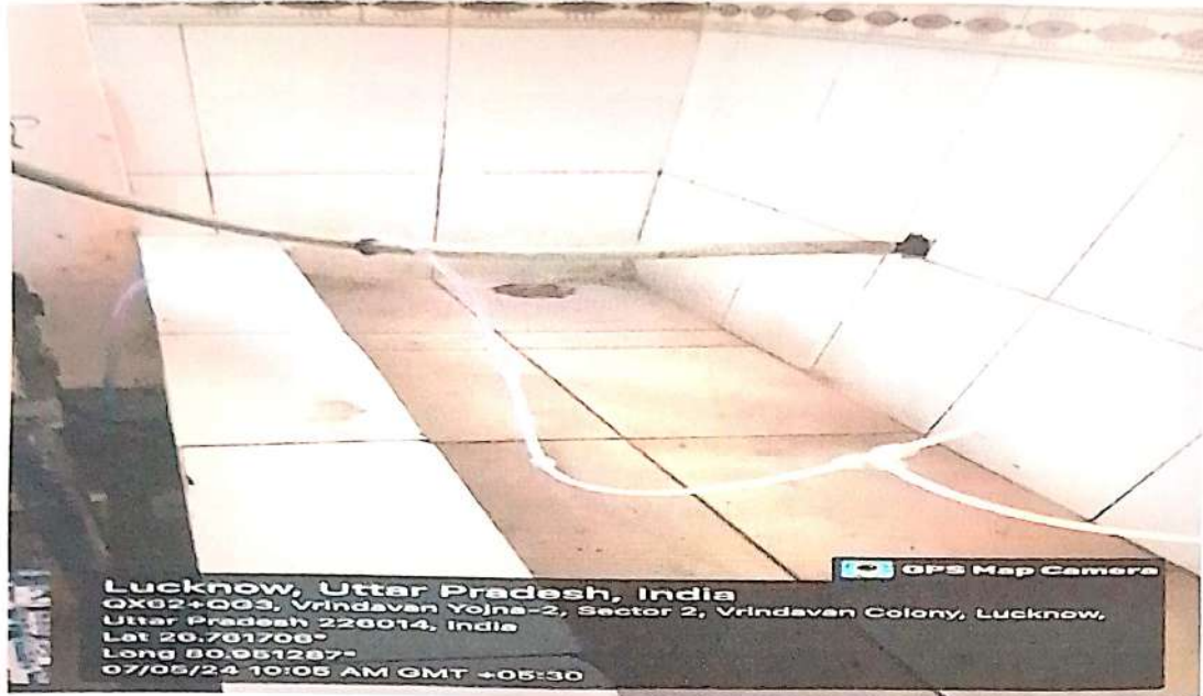
REUSE OF RO WASTE WATER SYSTEM
